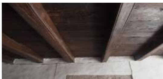
Picture 24. Structural wood of oak in traditional houses.
