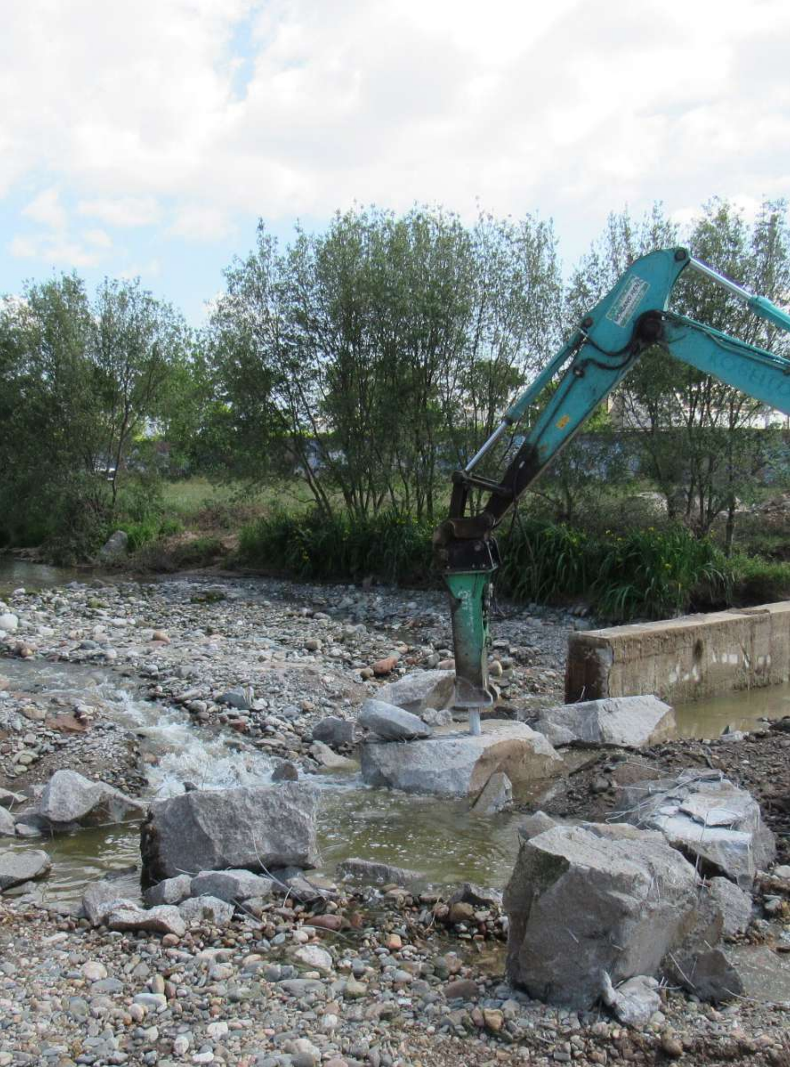
Restoration of sediment transport and lateral flooding with the removal of the canalization and an obsolete dam (Congost River in Granollers, Besòs basin) / Photo: Aprèn Serveis Ambientals
