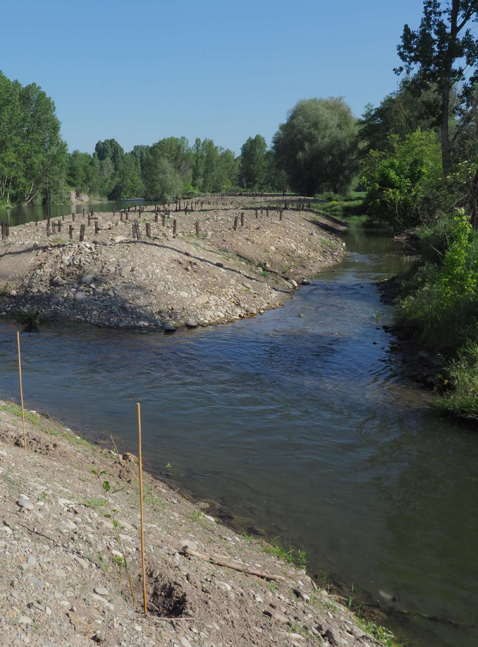
Recovery of flows in a minor arm of the river Ter, thanks to the restoration of the hydromorphological dynamics of sediments. Island of Les Gambires (Torelló, Osona county) / Photo: Jordi Camprodon.
